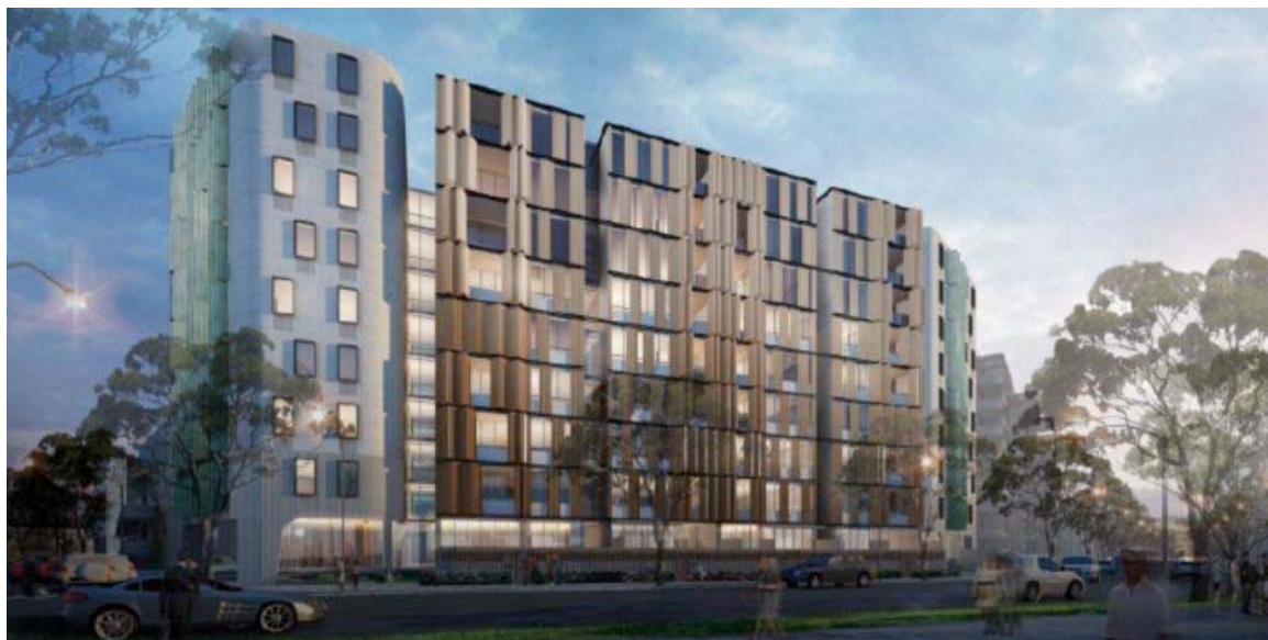
Figure 11: Building B viewed from Dalmeny Avenue.
