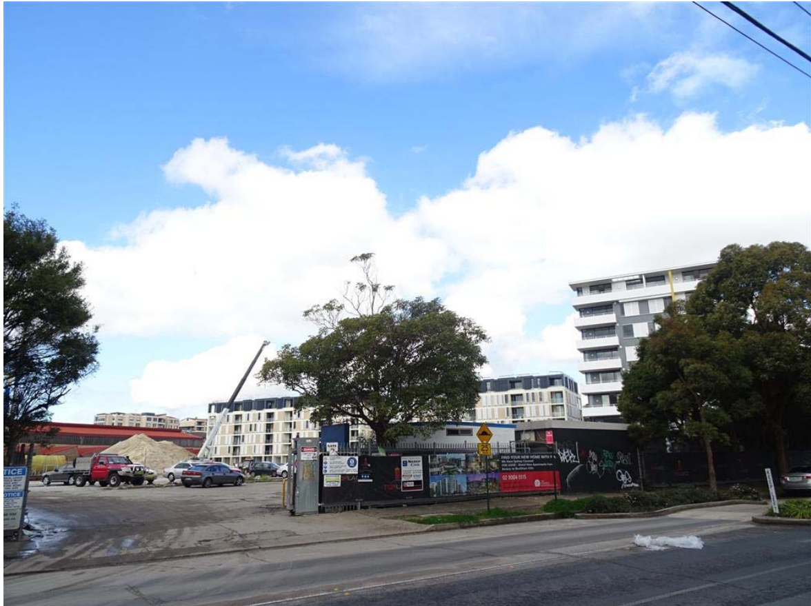
Figure 3: The site viewed from Dalmeny Avenue.
