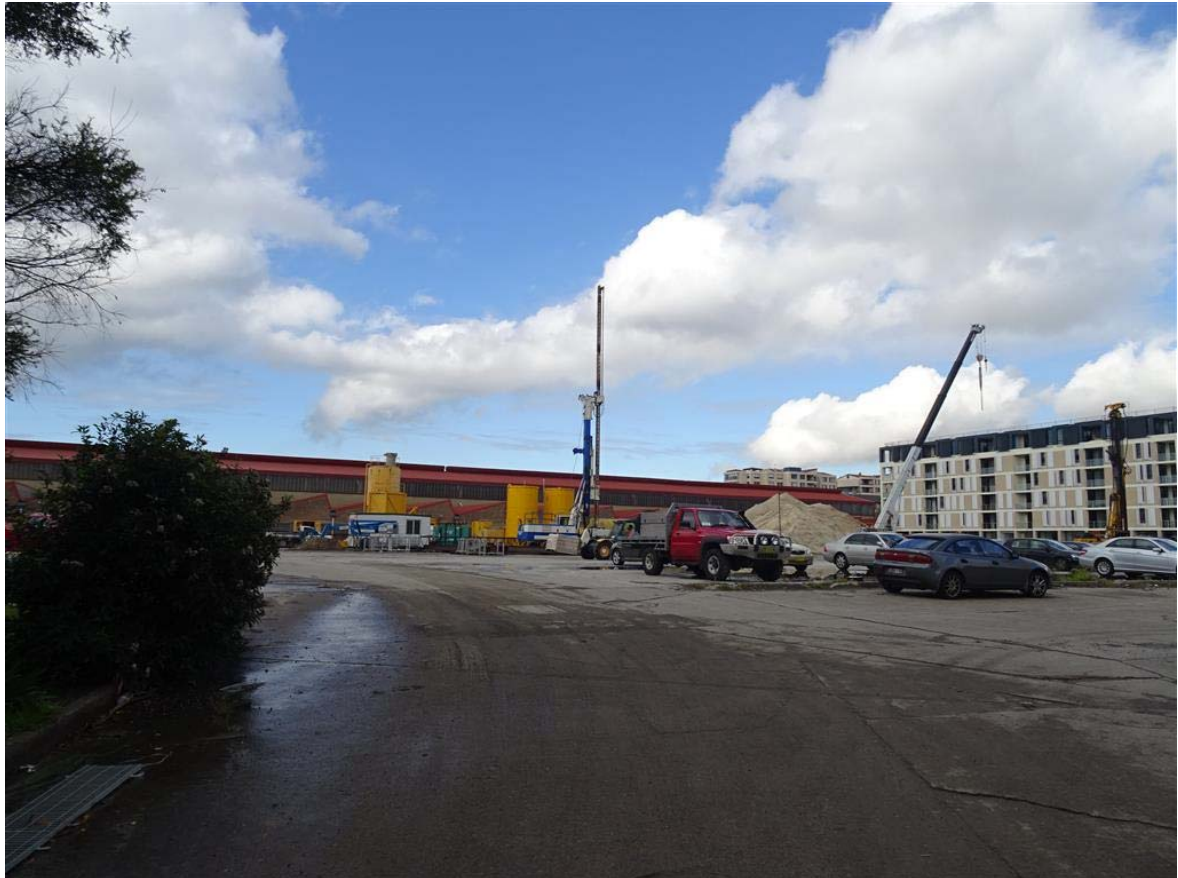
Figure 4: Looking east across the site.
